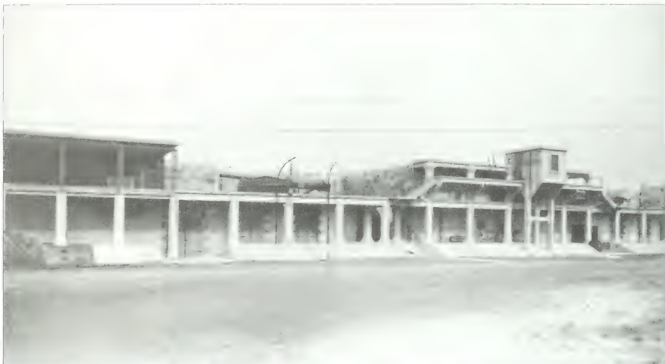
Figure 2.34. View looking southeast at Battery Granger, circa 1907. In 1907, Battery Granger was updated by extending platforms behind the guns for more convenient loading of ammunition. Additionally, an enclosed, concrete battery commander's station was added between the gun emplacements (Thomas Hoffman, Fort Hancock , Charleston, SC: Arcadia Publishing, 2007).
